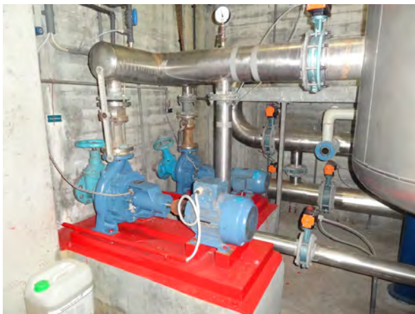
Filterpumpen
